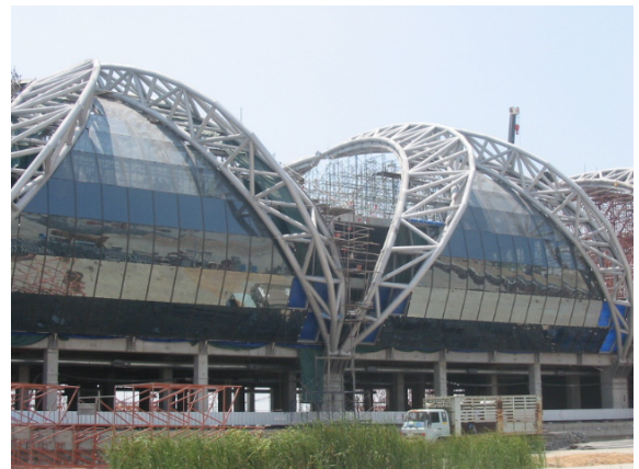
The airport consists of 208 'bays' made up of over 100,000 m 2 of pre-treated ClearShield glass
