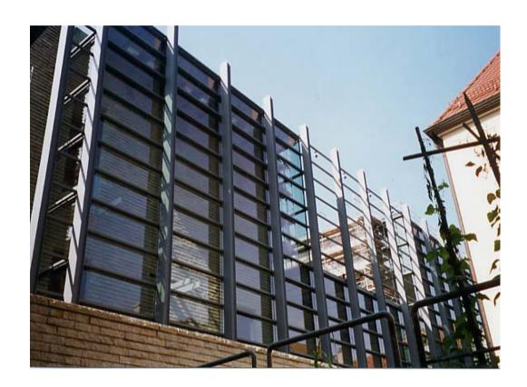
This museum opened In May 2001. Visionary Danish architect Henning Larsen of Copenhagen specified ClearShield for the high quality white glass supplied by Interpane. The glass used was 8mm special Ipasol Natura 6634 and a total 2,100m² of glass was protected with ClearShield. Contamination on the glass during construction was easily removed and reduced delays, thanks to ClearShield protection.
