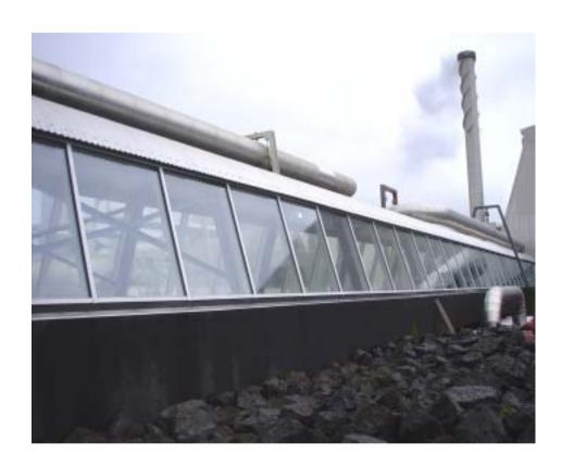
Despite frequent cleaning and the use of harsh chemicals, the building's glass would quickly become dirty again due to the extreme silica-rich environment. When the time came to replace the old, ordinary glass, some 1,000m² of new ClearShield glass was installed in 1994.
