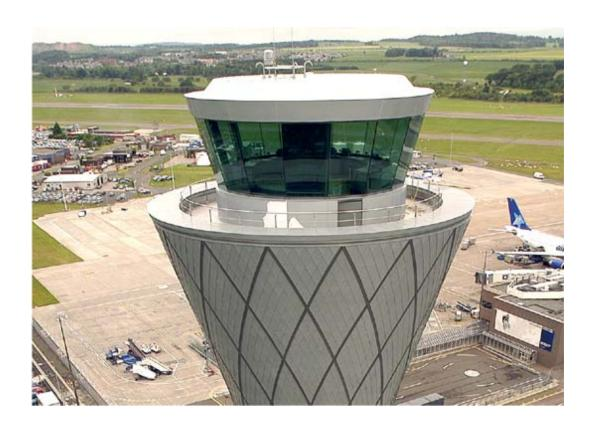
Edinburgh Airport is the eighth largest airport in the UK and a new control tower was completed in 2005. The lead contractor was recommended by a control tower design and build specialist to specify ClearShield to improve visibility for air traffic controllers as well as reduce maintenance needs.
