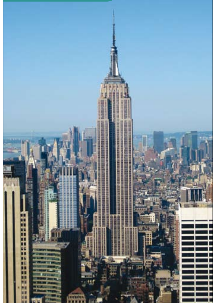
Empire State Building, New York City: On-site renovation only
