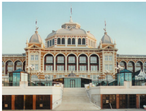
Roof glazing Kurhaus Hotel, Holland
