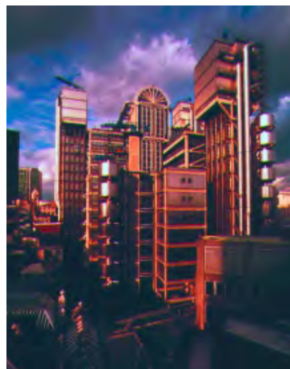
(below) Lloyds of London Building
