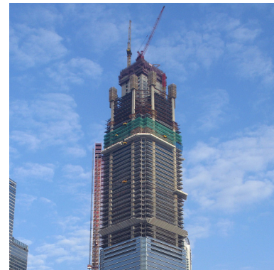
International Commerce Centre, Hong Kong
