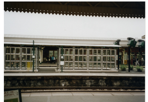
Platform glass Taunton Station, UK
