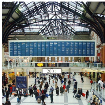
Roof glazing Liverpool Street Station, UK
