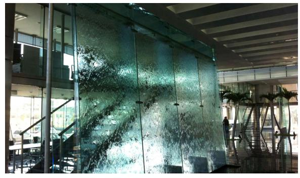
**The problem:** water running down the waterfalls is not filling all the glass surfaces at the lowest part of the glass, especially at the edges of the glass and hard to be pushed at the top part. The water is not covering the entire glass surface.
